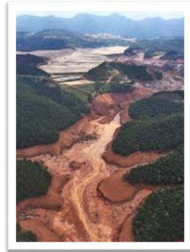
Fundão dam collapse
