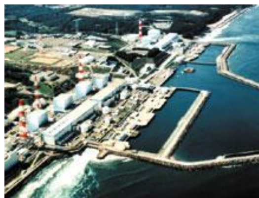
Image 1: The Fukushima Dai-ichi nuclear power plant with six reactors. Source: TEPCO
